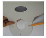
Ouse the mount to mark the pilot holes are required. Drill holes into the drywall and insert the drywall mounts.
