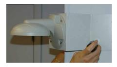
Mount the camera assembly to the corner of the wall, using wall mount anchors and machine screws.
