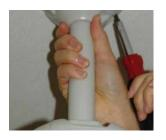
Use the mounting template to make pilot holes. Use the dry wall anchors and machine screws to attach the assembly to the wall
