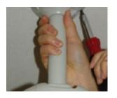
Use the mounting template to make pilot holes. Use the dry wall anchors and wood screws to attach the assembly to the wall
