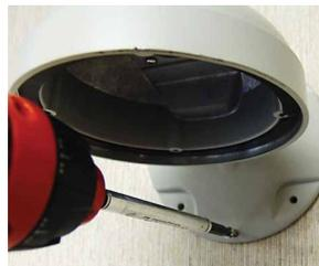
3. Use the mounting template to make pilot holes. Use the dry wall anchors and woods screws to attach the assembly.
