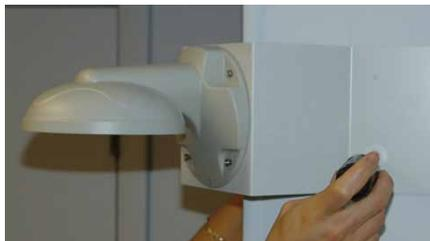
4. Mount the camera assembly to the corner of the wall, using wall mount anchors and machine screws.
