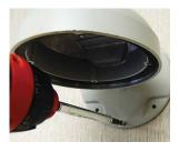
Use the mounting template to make pilot holes. Use the dry wall anchors and woods screws to attach the assembly.
