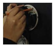
3 Use camera mounting template or your camera to mark the holes as required.
