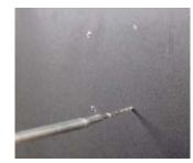
4 Drill holes into the drywall and insert the
