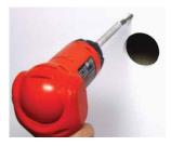
3 Drill holes into the drywall and insert the drywall mounts into the holes
