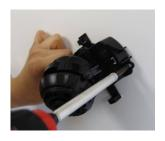
Pull wires through and make connections. Then, mount the camera to the wall using the included machine screws
