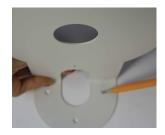
Use the mount to mark the pilot holes required. Drill holes into the drywall and insert the drywall mounts.
