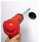
2 Drill holes into the drywall and insert the your camera to make holes as required. drywall mounts.
