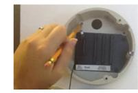
Use the camera's mounting template or your camera to make holes as required.
